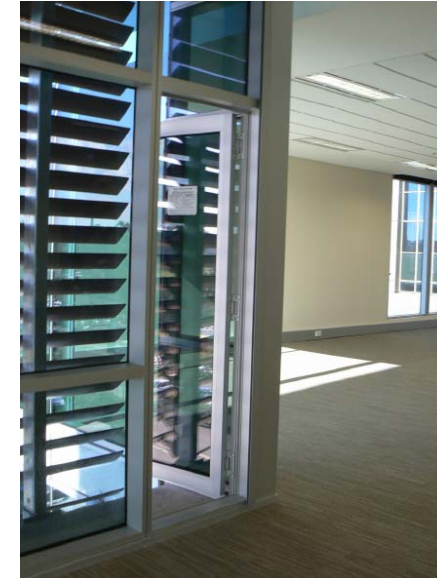
Above: Internal door to access Façade
